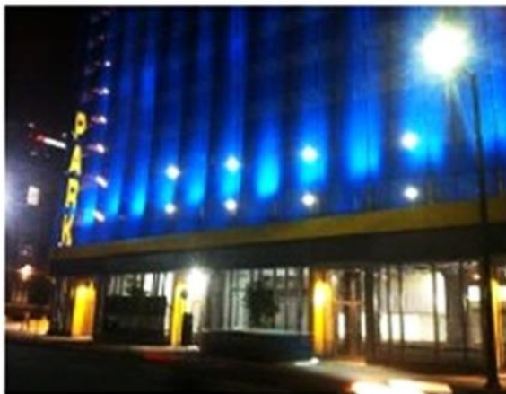
*ACTUAL PICTURE OF PARKING GARAGE*
